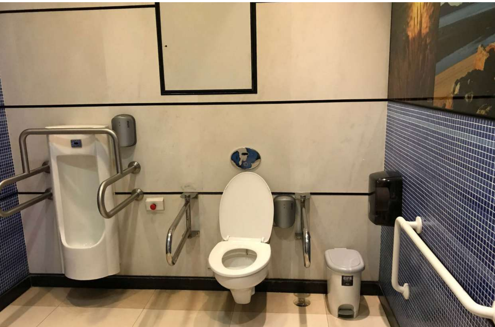
Image 4.19 Grab bars in the Accessible Washroom Photo Credits: Dr. Gaurav Raheja
