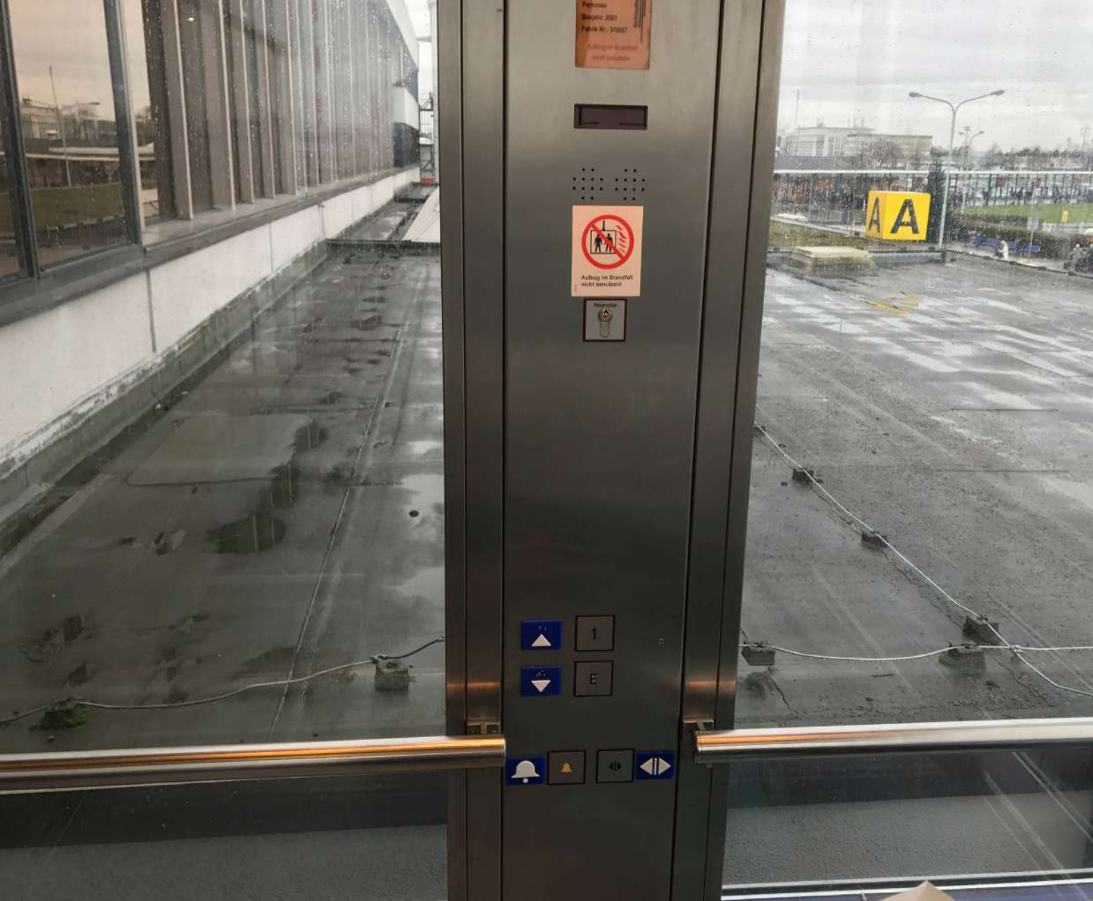
Image 4.10 Accessible control panel in the lift Photo Credits: Dr. Gaurav Raheja
