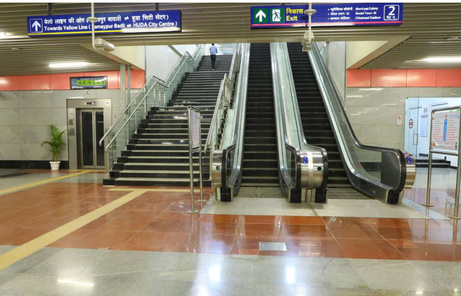
Image 6.21 Inclusive vertical circulation in train station enabled with Lift, staircase and escalator Photo Credits: DMRC
