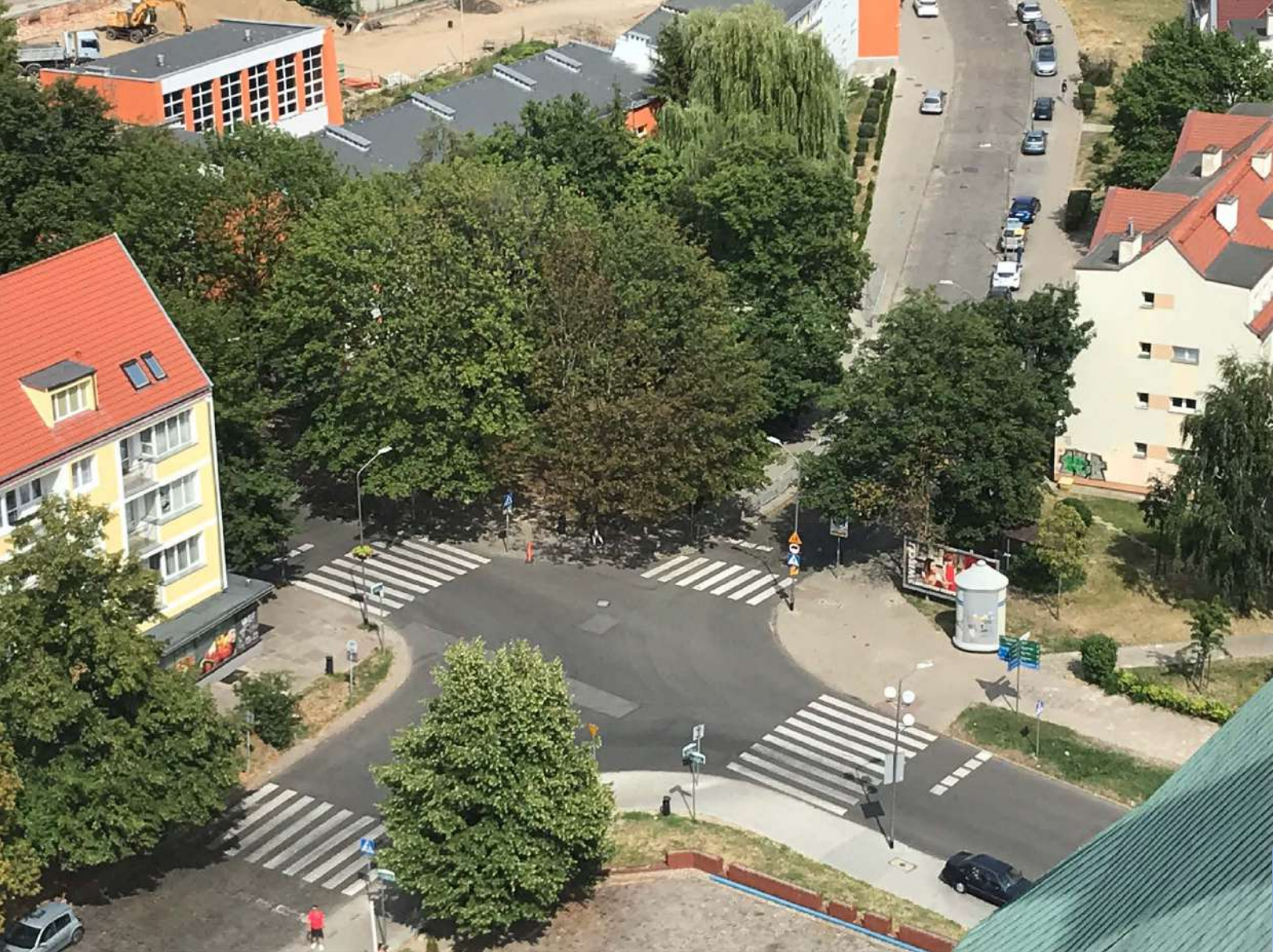
Image 3.14 Accessible road intersection with pedestrian crossing Photo Credits: Dr. Gaurav Raheja
