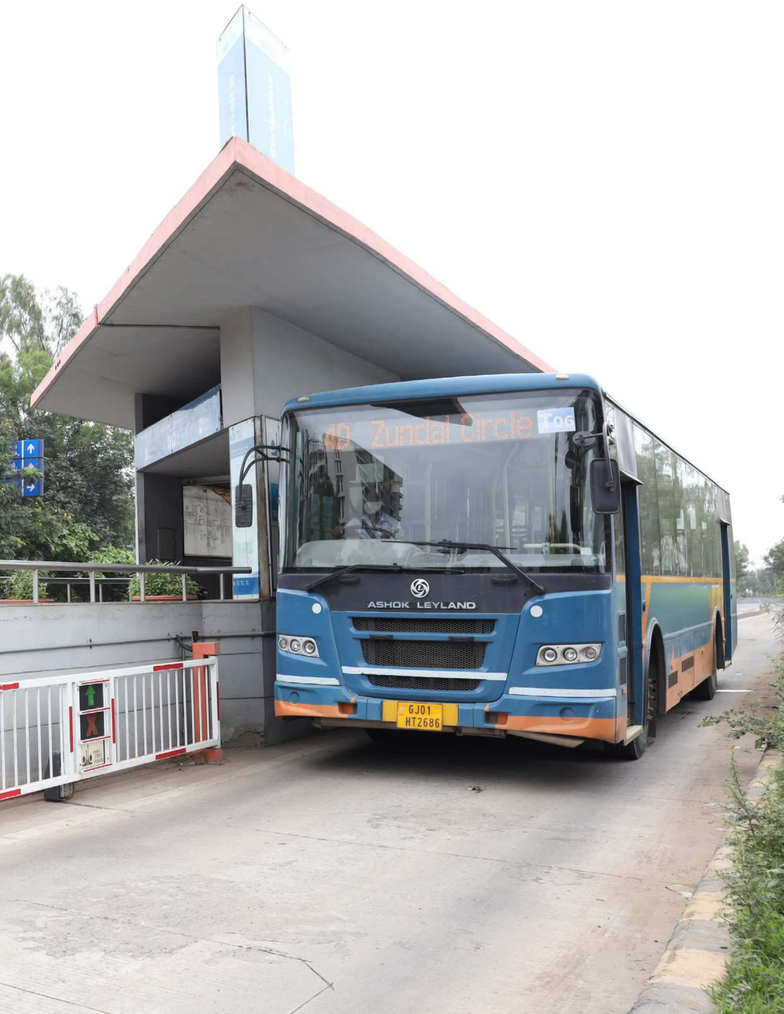
Image 6.14 Accessible bus station with level approach Photo Credits: CPWD
