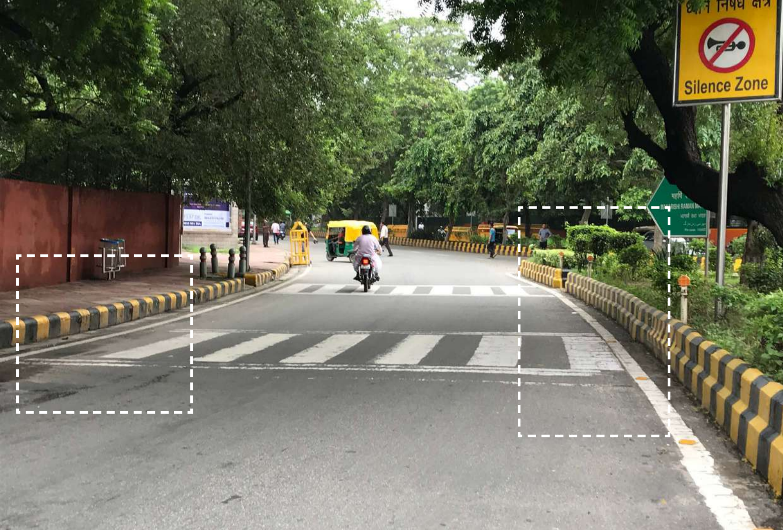
Image 2.27 High kerbs and absence of kerb ramps near zebra crossing
