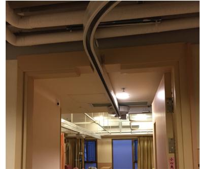
*[Fig. 7A.4] Additional space may be needed to accommodate a patient lifting equipment so the provision should be considered at early planning stage.*
