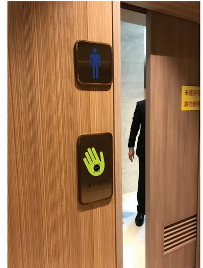
*[Fig. C3.1] A sliding door is fitted with hands-free operator that helps the elderly to open/close the door easily.*
