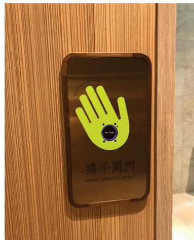
*[Fig. D5.1] This “Wave Hand to Open” door operator incorporates intuitive graphic design to guide the users to operate the motion sensor.*
