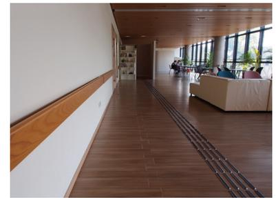
*[Fig.D2.2] Handrails in high visual contrast against the background can help individuals with visual impairment to locate the handrails.*
