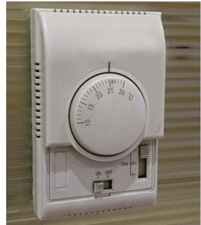
*[Fig. C5.1] A thermostat with an user friendly dial allows easy adjustment of room temperature*
