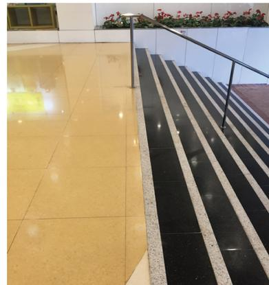
*[Fig. B5.2] Edges of landing and steps should be highlighted to warn users of changes in floor surface level.*
