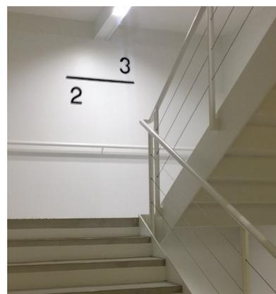
*[Fig. B5.3] Appropriate sign that identifies floor level should be provided at landing.*
