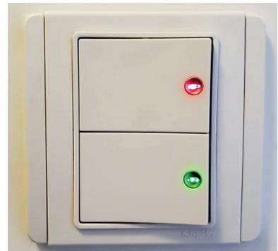
*[Fig. 7A.5] An example of a light switch with LED indicator that can help the elderly to locate the light switch in the dark.*
