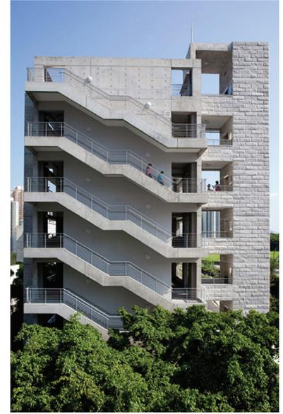
*[Fig. 7F.1] - Open staircase and lift lobby can enhance visual connection and maximize visibility and allow early detection of accidents.*
